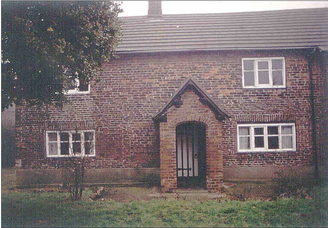
Figure 130: The western elevation of Wigsey Farmhouse.
