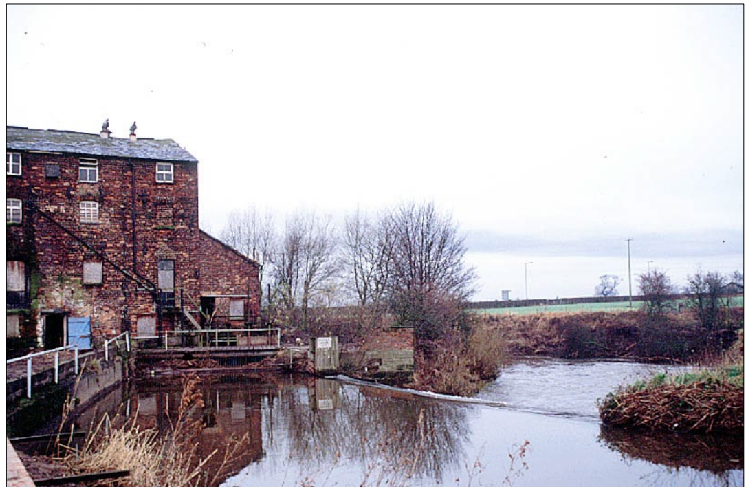
Figure 148: The western and southern elevations of Warburton Corn Mill, 1999.
