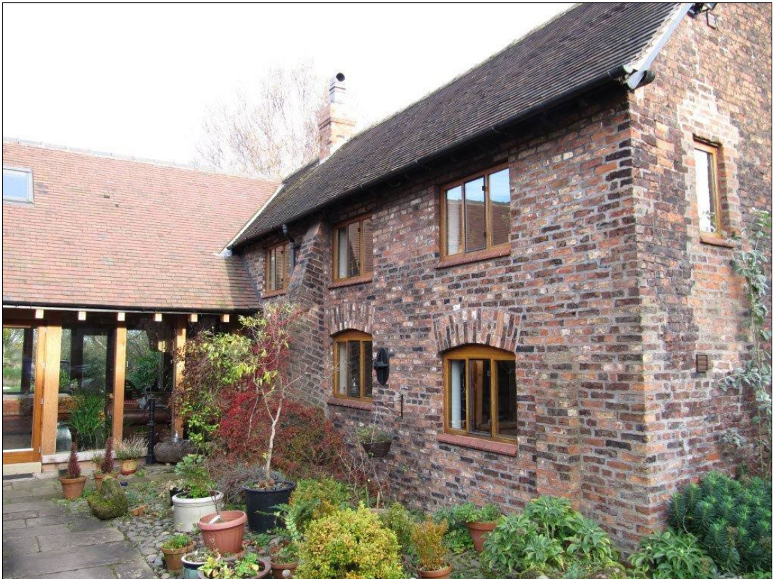
Figure 98: Onion Farmhouse looking north, 2023.
