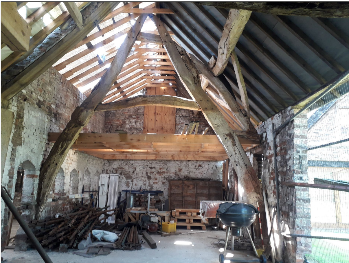
Figure 141: The cruck trusses at Heathlands Farm barn.
