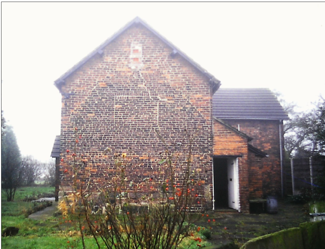
Figure 131: The northern gable of Wigsey Farmhouse showing the earlier roof line and blocked window.
