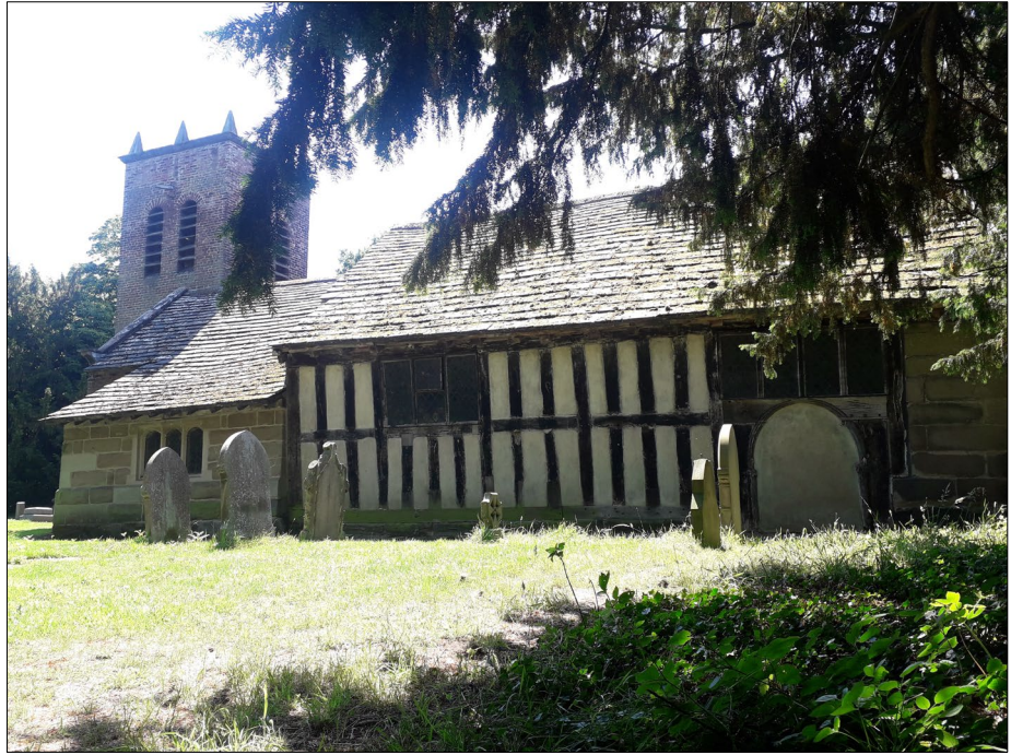
Figure 92: St Werburgh's old church northern elevation and tower.
