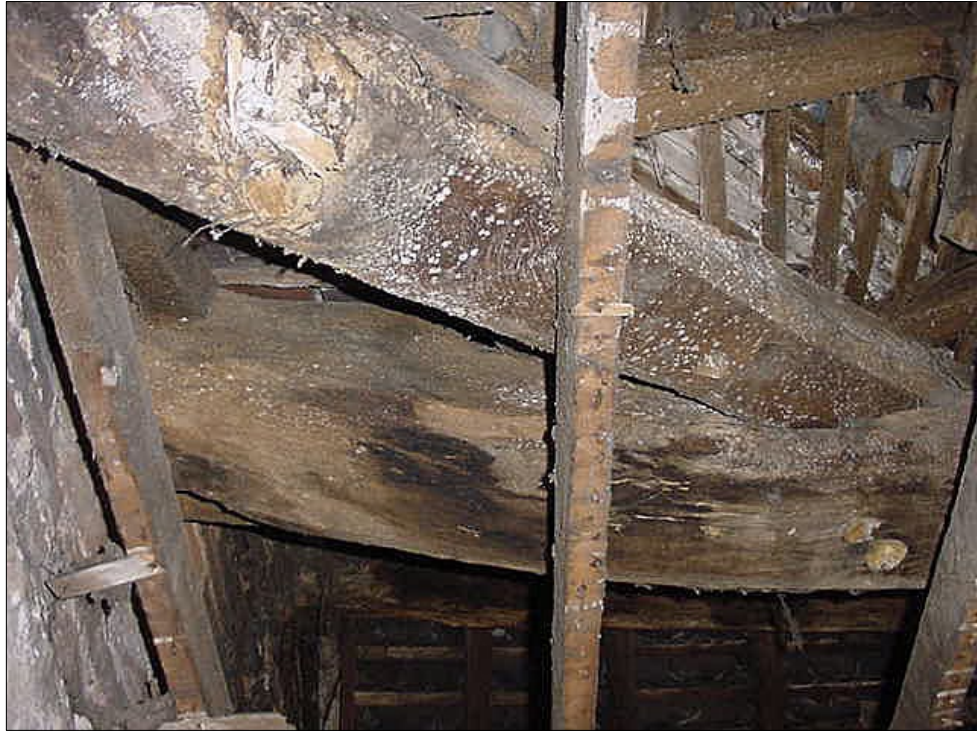
Figure 119: Re-used cruck blades in the roof at Paddock Lake Farmhouse.
