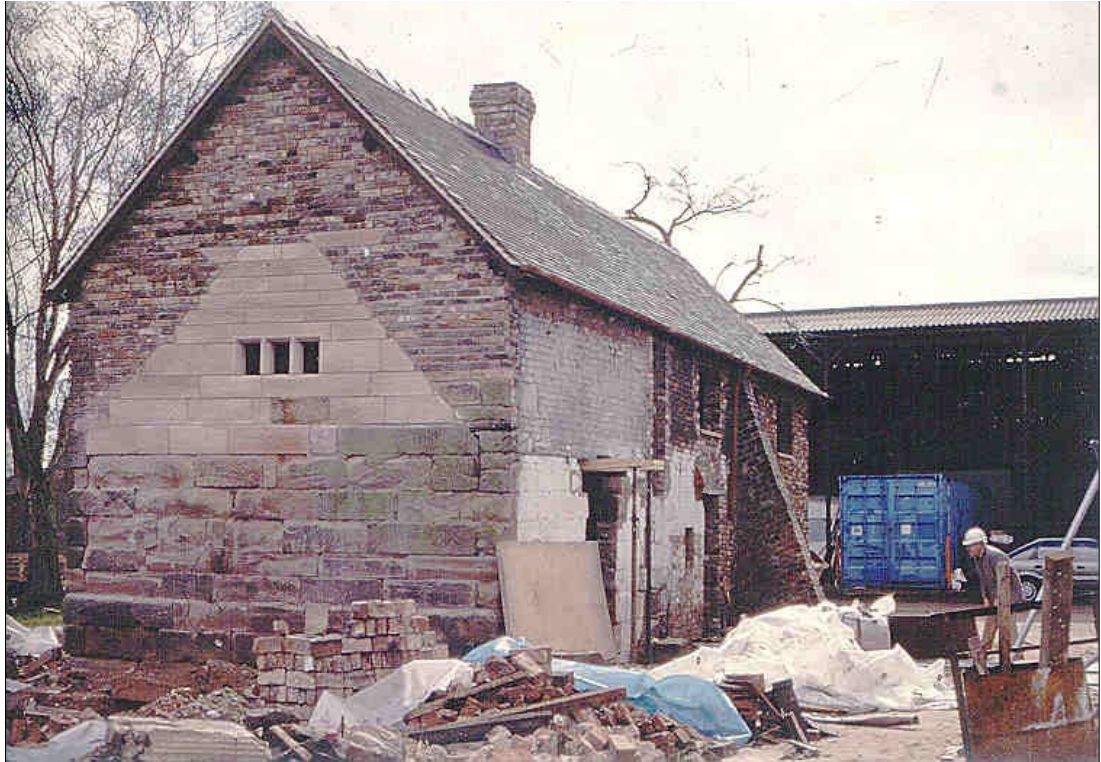
Figure 99: Onion Farmhouse looking south before restoration in 1996.
