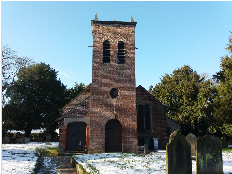
Figure 90: St Werburgh's old church eastern elevation and tower.
