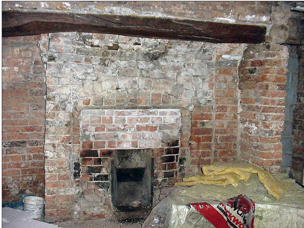
Figure 120: Inglenook fireplace at Paddock Lake Farmhouse.
