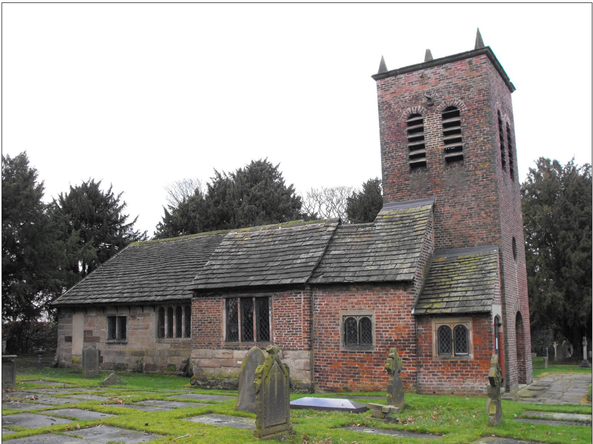
Figure 91: St Werburgh's old church southern elevation and tower.
