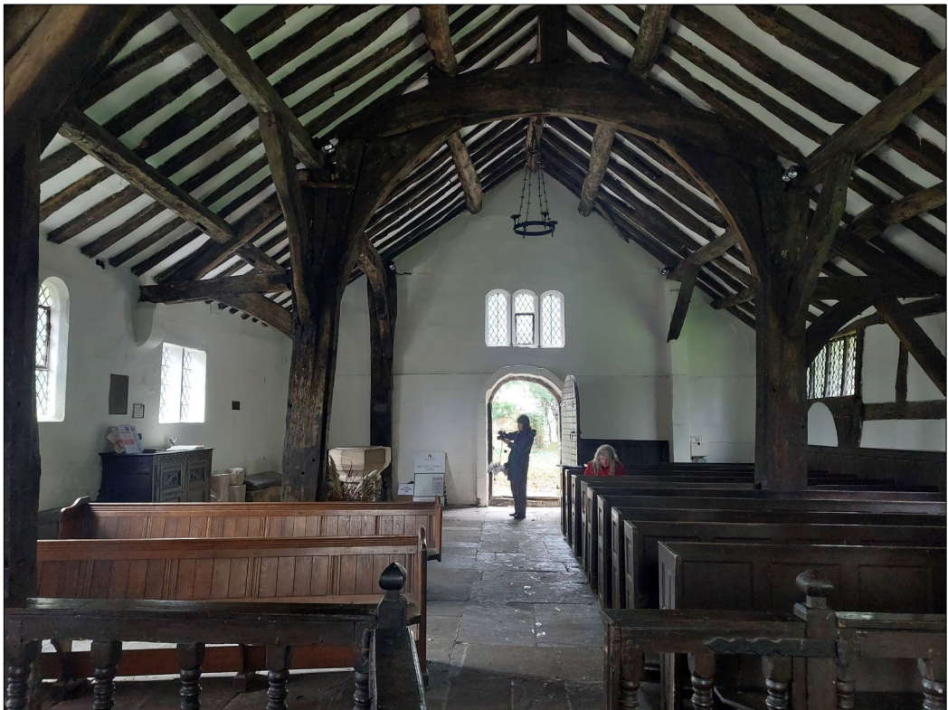
Figure 95: St Werburgh's old church interior looking west.
