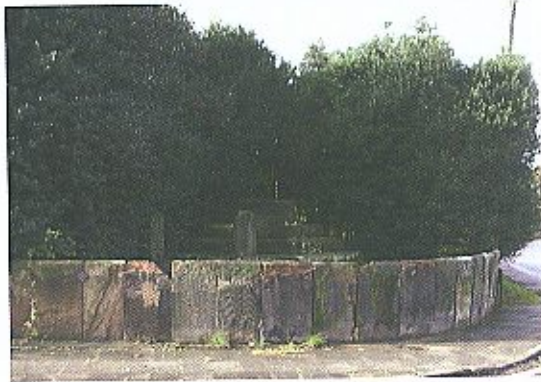
The wall which surrounds the cross base is made of slabs of local sandstone held together by iron cramps.
