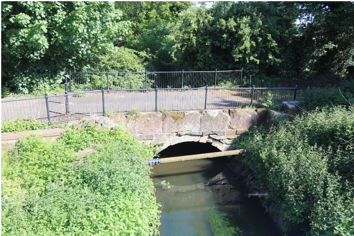
The old bridge carrying Warburton Lane over Red Brook.
