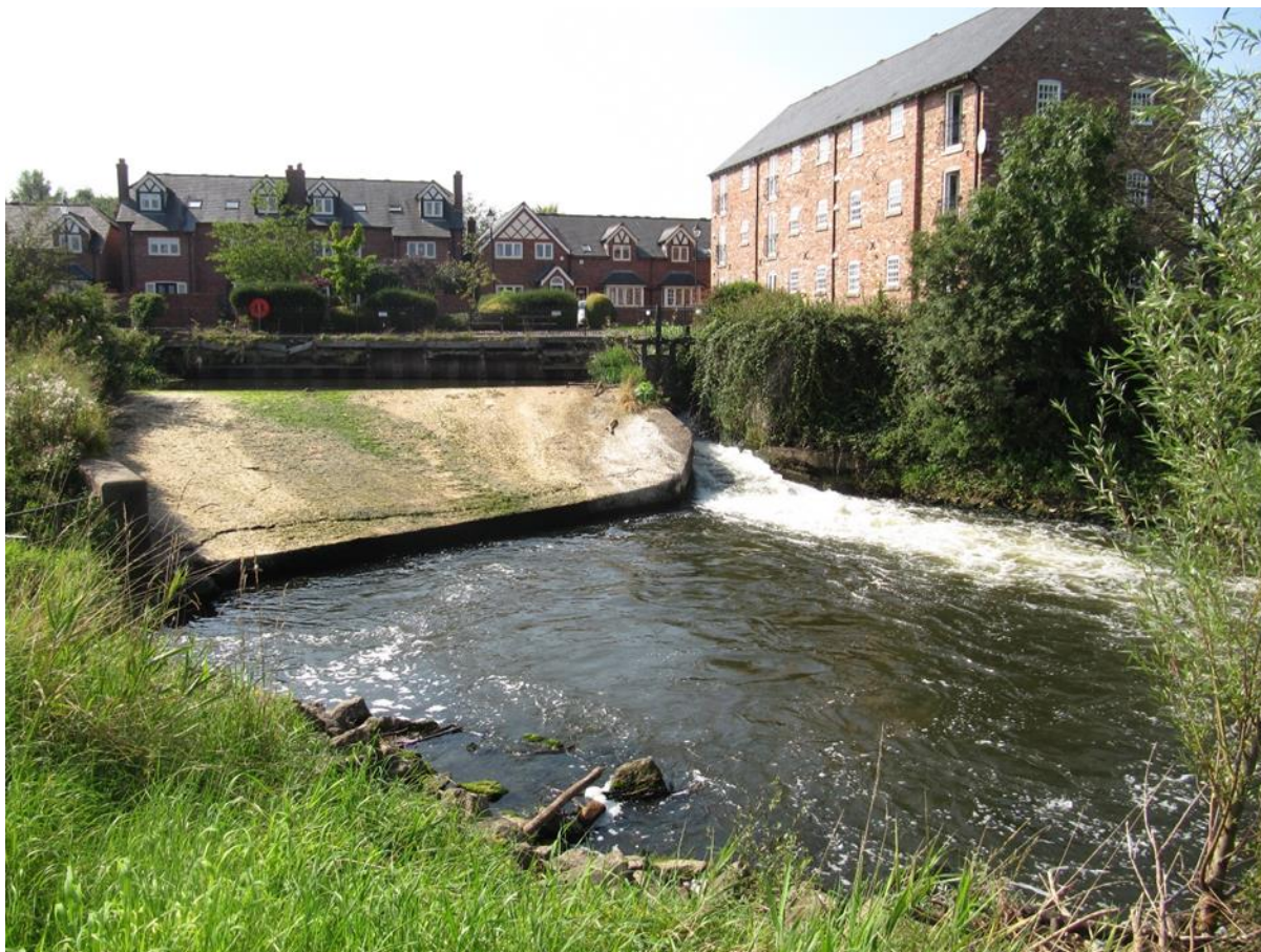
Above; the weir and modern flats replicating the old Warburton Mill.
